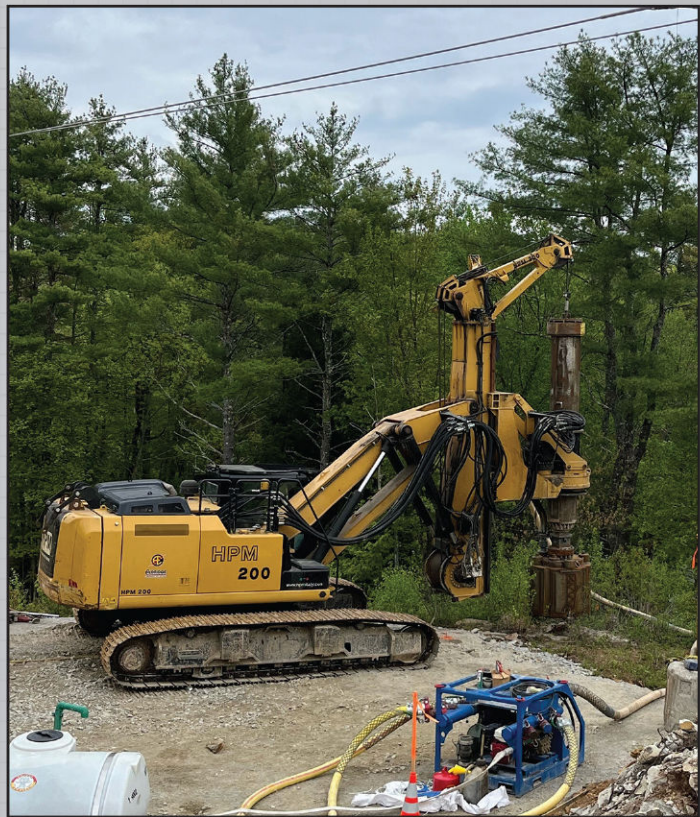
48" XLP transmission project on low headroom drill.
