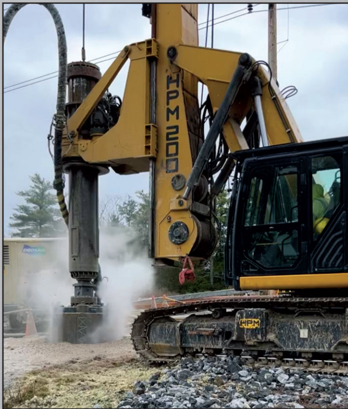
48" XLP transmission project on low headroom drill.
